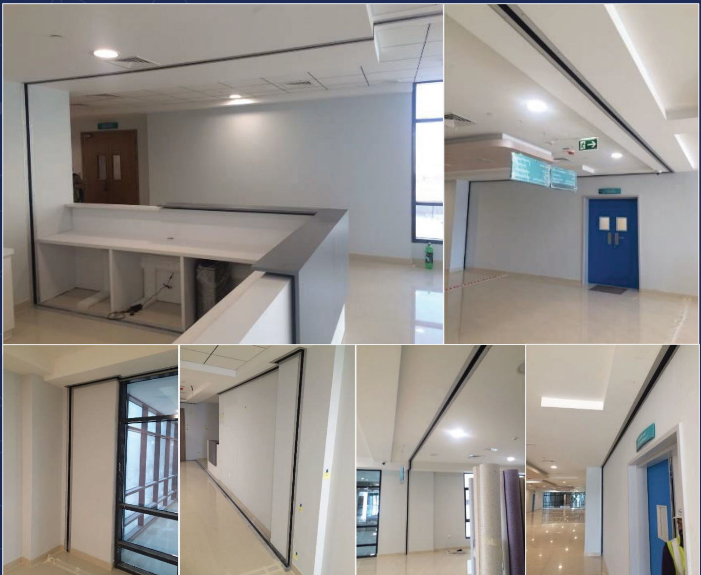
Floor Expansion Joint
